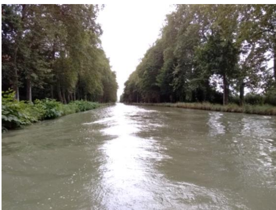
Figure 5 : aval de la station
