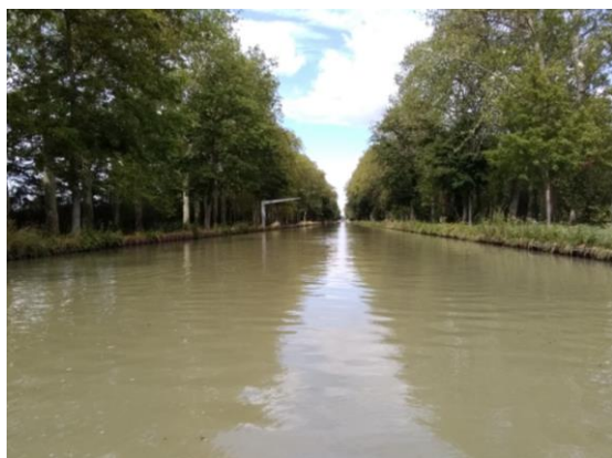
Figure 4 : amont de la station
